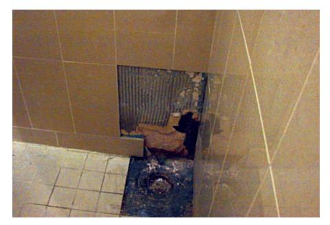
This was one of many showers which had a glass mat backerboard placed in the bottom of the mortar. The wall was saturated approximately 24" up the wall. As it was in front of the shower pan, water was being retained and strange growths were appearing in the grout joints.
