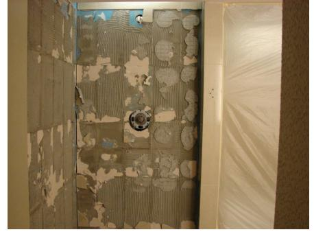
Some jobs leave me at a loss for words. This one-year-old project has waterproofed drywall; however, the joints were not taped and left open. The tile was then spot mounted to the wall and collected water through the grout, which was promptly dispatched to the kitchen ceiling below.
