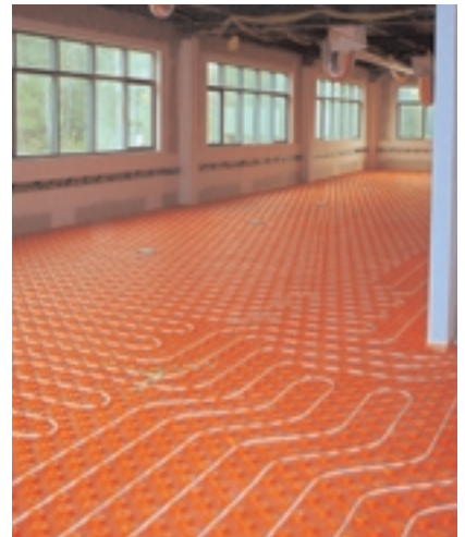
▲ Left: Geothermal Drill Right: Geothermal water tubes
