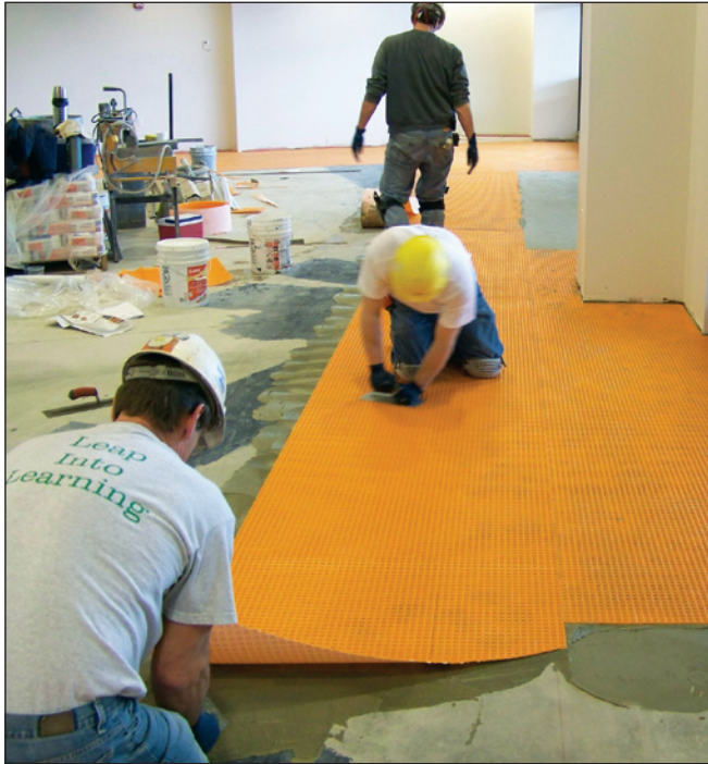
Uncoupling membrane application at Providence Park Hospital. The system's specification helped yield the necessary flexibility for placing movement joints.
